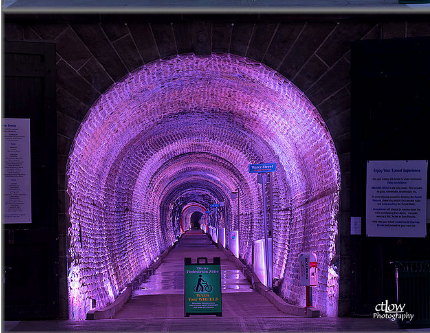
That day, the tunnel opened at 6 a.m. - this of course is before and after. You can't do a completely straight-on view, because it has a little crook at the north (far) end.
